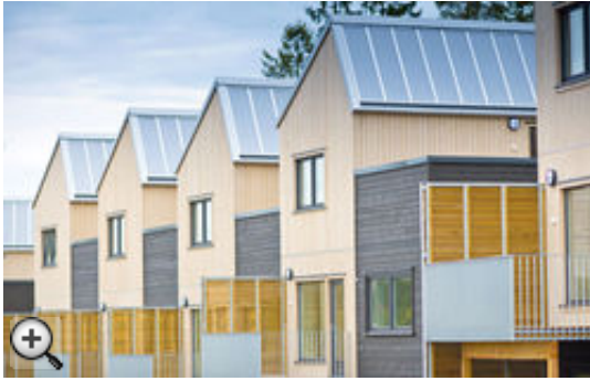
Solar collectors with extruded PPS absorbers (© JKU Austria/H. Kicker)
